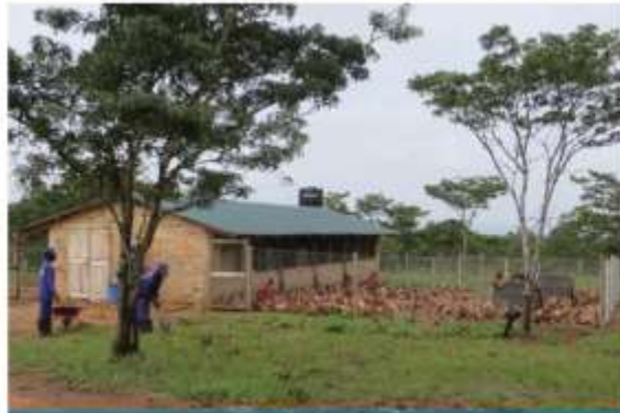
Training centre poultry houses
